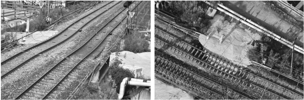
Figure 1. Deformation of the railways [4]. Figure 2. Aerial picture of the incident [4].
